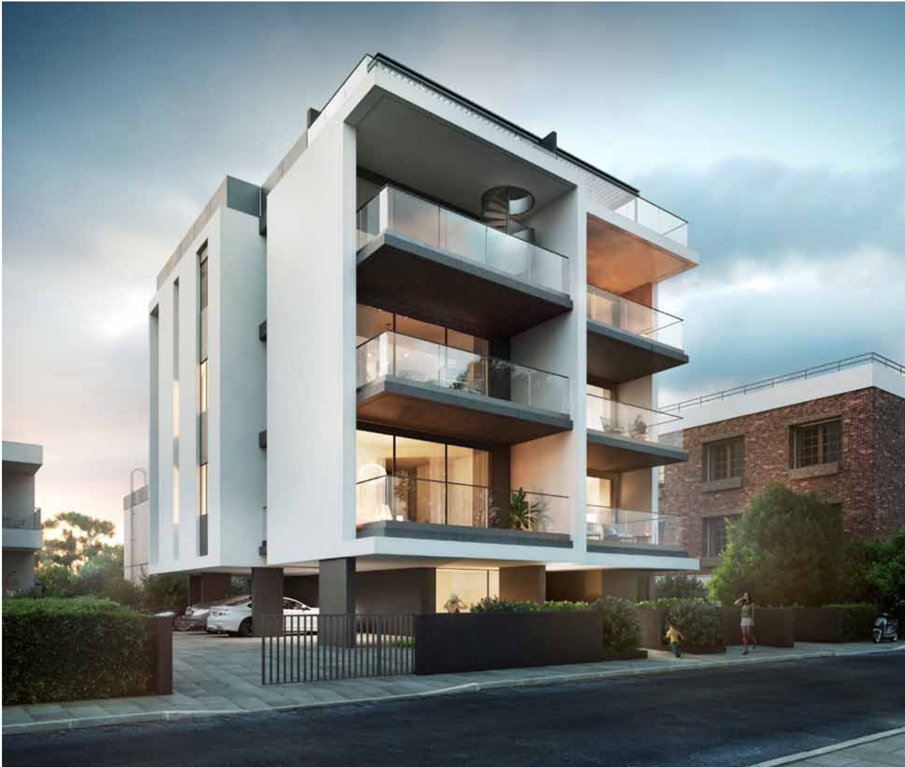
6/SEAFORD HOUSE/A PROJECT BY bbf®
